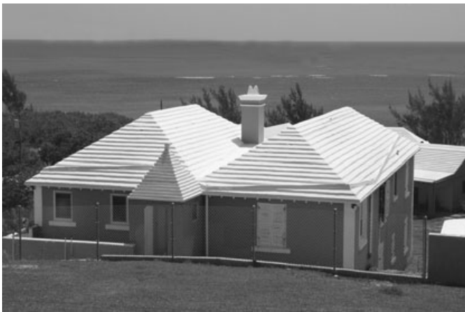
FIGURE 3. Photograph of a Bermuda Roof. Bermuda roofs are coated in an approved white paint which is usually cement-based. Gutters or “glides” are positioned close to the roof edge, achieving 80% coverage (as catchment) of the total roof area.
